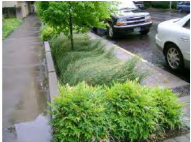
Planters as dividers between travel lanes and sidewalk
