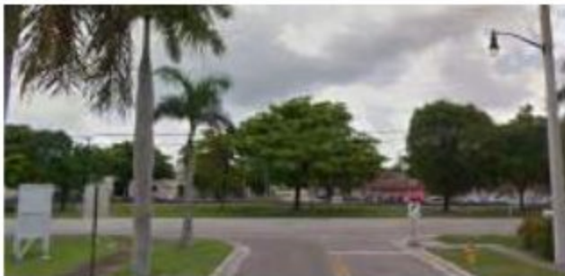
Dixie Hwy and Foster Road Intersection- Current Condition
