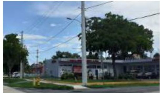
SW 11th Street & S Dixie Highway
