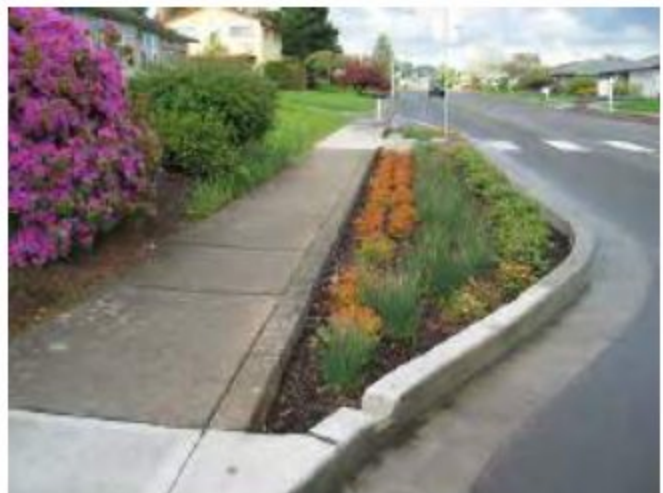
Stormwater curb extension
